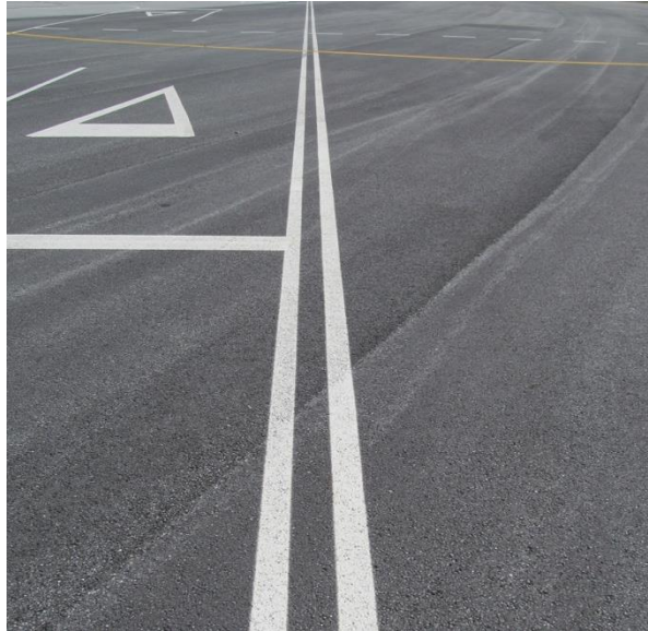
16-12 – Demarcation between the apron service road and apron taxiway
