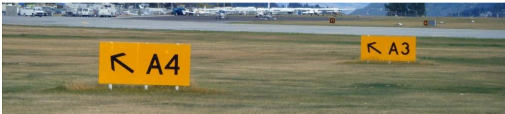
16-21 - Taxiway Direction Signs
