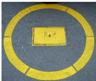
16-7 - Fire Hydrant marking
