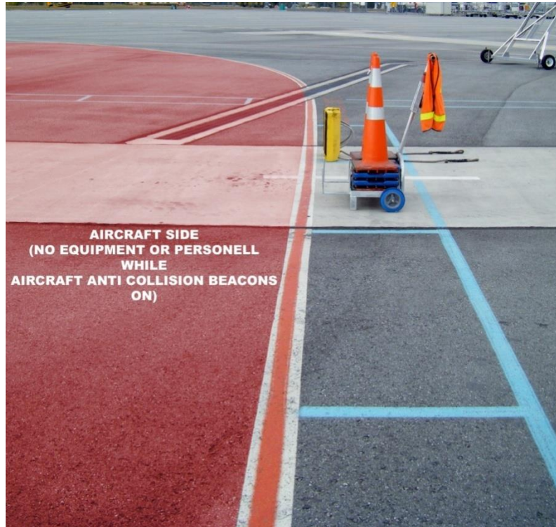
16-6 - Equipment Storage Limit Line
